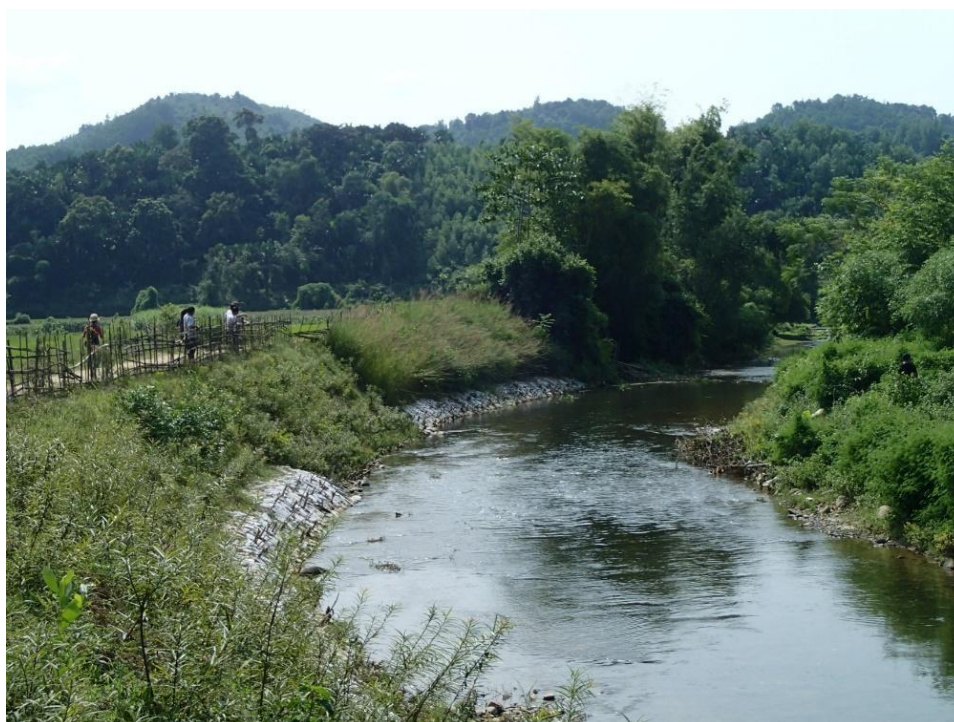
Figure 3.8: River bank restoration with native species, Son La, Vietnam
