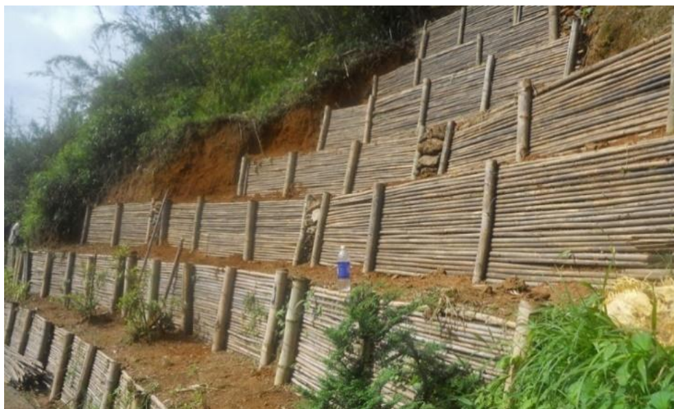
Figure 3.9: Live fencing, here utilizing local bamboo
